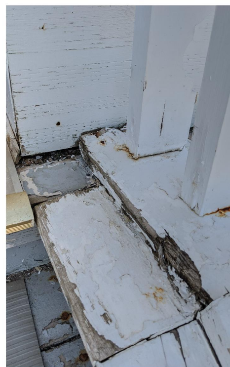
Railing base at the top of the stairs
